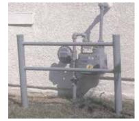
The Industrial Guard Post (left) is a medium duty barrier and the Residential Guard Rail (right) is a light duty barrier. Both are used to protect meter sets and/or regulator stations from vehicular traffic. The above ground portion of both is coated with a minimum of 2.5 mils polyester fusion coating.
